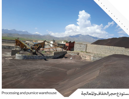
Processing and pumice warehouse
