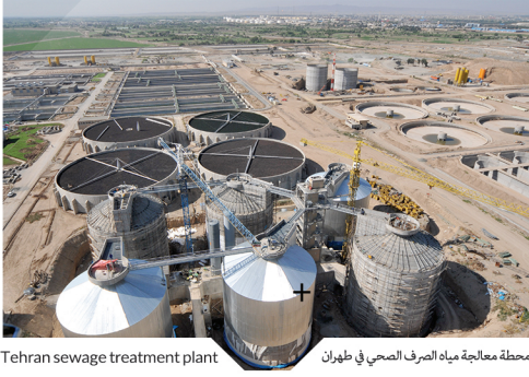
Tehran sewage treatment plant
